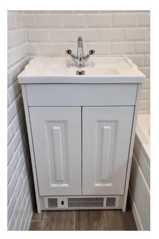
The vanity unit I ordered from Victoria Plumbing had a plinth the perfect size, this meant after studying the dimensions from Thermix I could cut a letterbox type opening, mounting the unit and the front grill would sit perfectly in the space.
